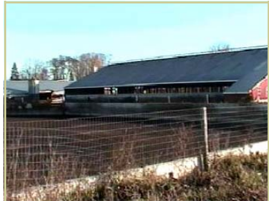
The recently updated and expanded waste storage facility.
