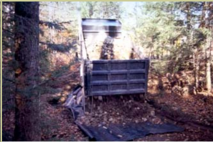
Ben Lorenson is a participant in the Forest Land Erosion Control EQIP. We helped him fix his woods road to reduce soil erosion.
