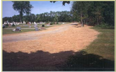
The newly seeded and mulched waterway at Morse's Corner Cemetery in Corinna
