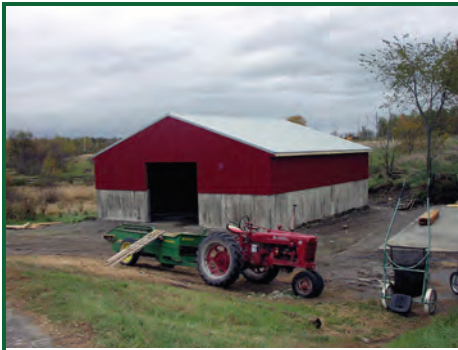
Roofed manure storage structures are now being used in areas where ground and surface water cannot be protected adequately.
