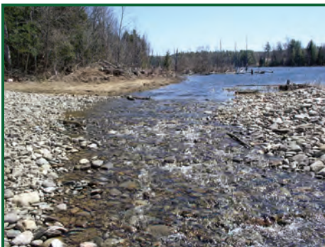
New rock-lined irrigation pond outlet.
