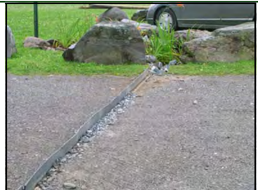
This rubber razor at Lakeside Landing diverts stormwater runoff into a rain garden rather than letting it flow down the boat ramp directly into Pushaw Lake.
