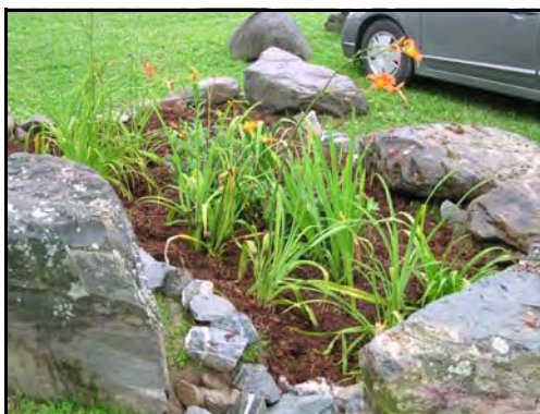
This rain garden was installed at Lakeside Landing to filter rain water that flows from the rubber razor.
