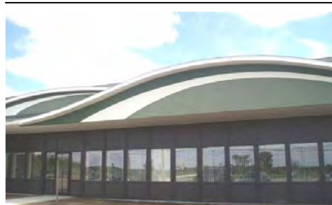
Our new office is located at 1423 Broadway in Bangor.
