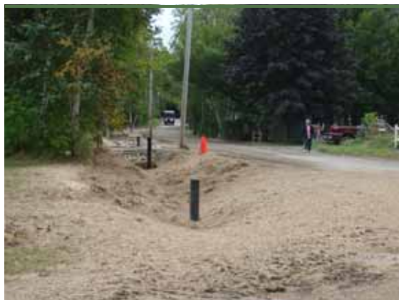
Upgraded drainage system on Woodland Ave in Old Town.
