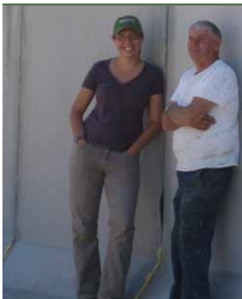
Heidi Bunn and Dennis Murphy, Sr. supervising construction on a manure storage facility.
