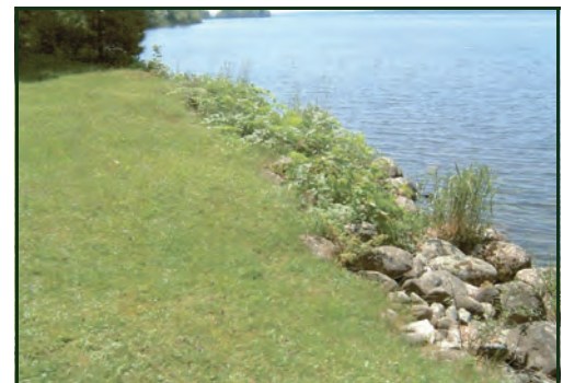
The site before the buffer installation.
